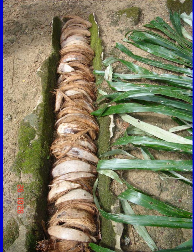
COCONUT HUSK PACKED DRAINS
